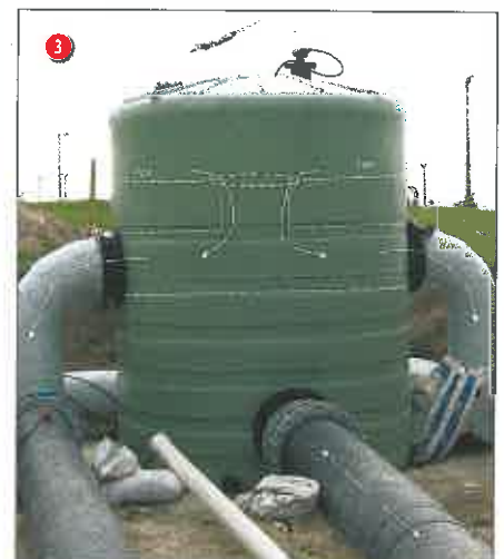
3 Photo 3: The BPS Famsys HDPE surge tank (before excavation backfill) c/w 450 NB HDPE inflow/outflow (surge) pipe and 400 NB GRP overflow / pressure relief pipework – normally dry (no signal from flow detector), but able to carry up to 0,5 cumec feed from internal 600 mm ND (variable elevation setting) drop-inlet spillway
